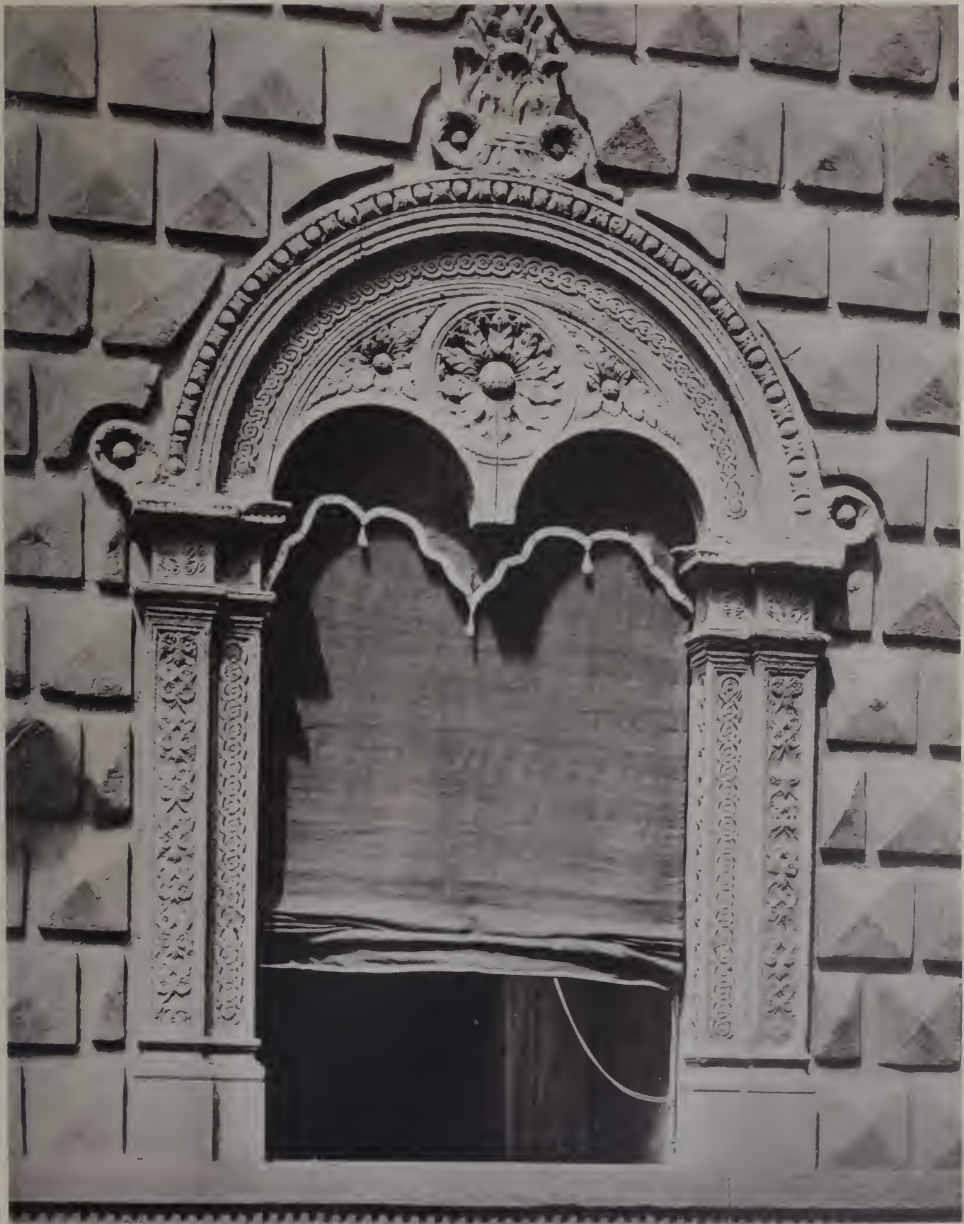
BOLOGNA. DETAIL OF WINDOW, PALAZZO BEV LAQUA
